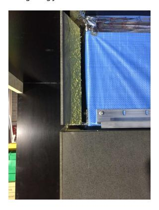
41) The top course below an eave or soffit requires brackets to be used in vertical joints.
