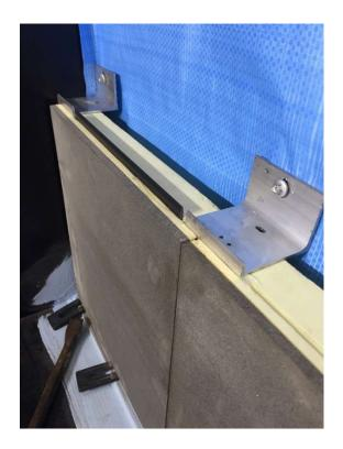
9) External corners may be one-piece premade units (as seen on top in the picture below) or made up with standard blocks on site with a 'quirk mitre' detail.
