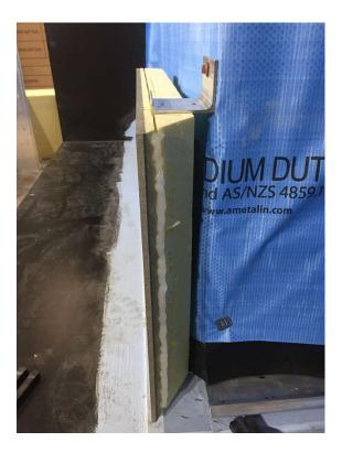
11) The second block is fixed into place leaving an internal 90 degree angle quirk detail with even side length each way on the external corner.
