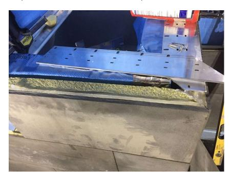
19) Should the wall continue above a box gutter or flashing to a roof the Reveal Rail extrusion is fixed to the structure ensuring the bottom of the rail laps a minimum of 10mm onto the upstand of the gutter or flashing to ensure any water exiting the weep holes is caught.
