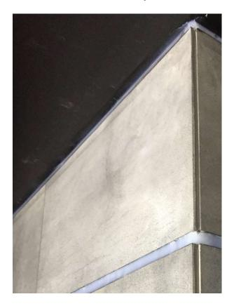
The product is weatherproof if installed according to the above instructions, even though the nominal 3mm joint will appear to be open once finished. This 'open' joint may be caulked or grouted in a complementary colour once the wall is finished without affecting its performance. Should a traditional 'mortar joint' be desired a bevel is machined on the blocks and flexible sanded grout used to fill the joint, giving it the appearance of having been laid with mortar as seen below.
