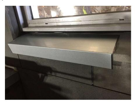
49) The junctions between windows, doors, sills, blocks and Reveal extrusions should be sealed.
