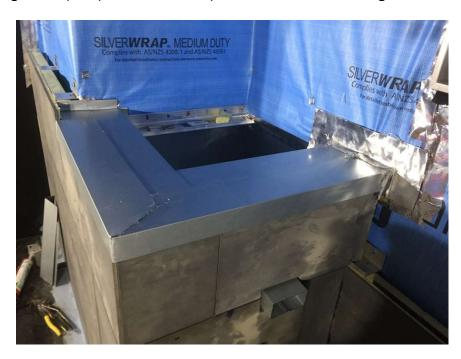
21) Where stone will be running over a parapet that intersects a wall the flashing should extend to the structural wall and turn up a minimum of 30mm.
