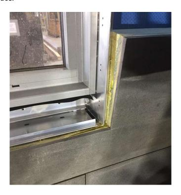
29) Once it is at the right height the block can be pushed up against the Reveal extrusion fitted to the side of the window to ensure a tight seal and then fixed in place with a bracket.
