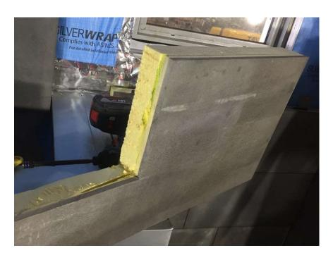
27) The portion of the block that will fit on the wall below the Reveal extrusion that will support the sill should have the backing board cut back at an angle to ensure it will not impede fitting of the block.
