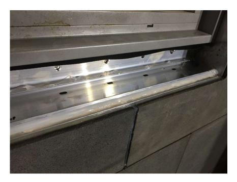
46) Place the sill below the window and lower the back edge onto the support ledge at the back of the Reveal extrusion. This will keep the back up and maintain the angle of the sill as you lower it onto the locating flange on the bottom of the Reveal extrusion.
