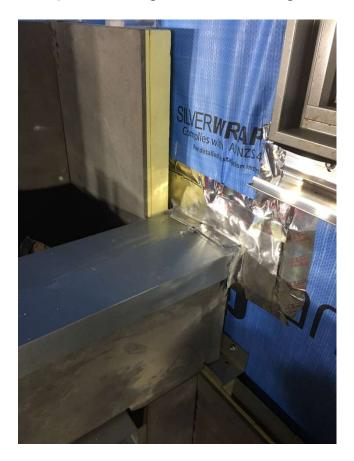
23) Windows should have flashing applied according to manufacturers' instructions and sealant should be applied between it and sarking below.
