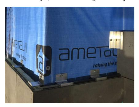
37) Brackets may be used in vertical configuration as shown below. When working between two fixed points it is best to leave the corner block to be the last one set in place.
