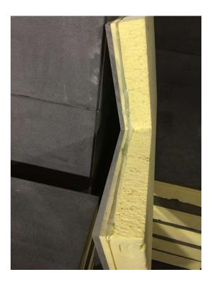
34) Sealant may also be applied to Reveal extrusion locating flanges prior to installation of the block.
