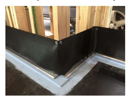
4) Sarking is then fixed to the frame according to manufacturer's directions taking care to ensure it overlaps the dampcourse by a minimum of 150mm.
