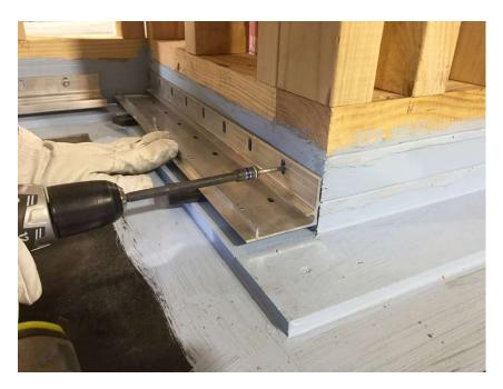
2) Care should be taken to ensure each rail is closely fitted to the next, and a maximum gap between any two extrusions of 10mm is allowed for expansion joints.
