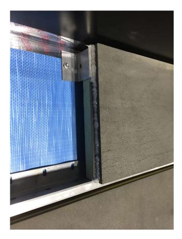
43) Horizontal and vertical expansion joints and anywhere that the system abuts other materials should have a minimum 10mm gap that is to be filled with backing rod before sealant is applied. Low-tack masking tape is used to protect the surface of the stone prior to sealant being applied. The tape should be removed as soon as sealant has been applied to ensure no residue is left on the face.
