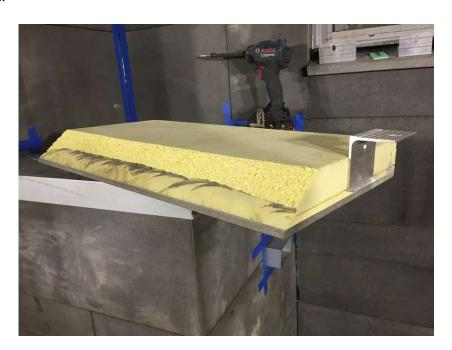
52) The block is then fitted to the Reveal extrusion already in place and the bracket fixed to frame.
