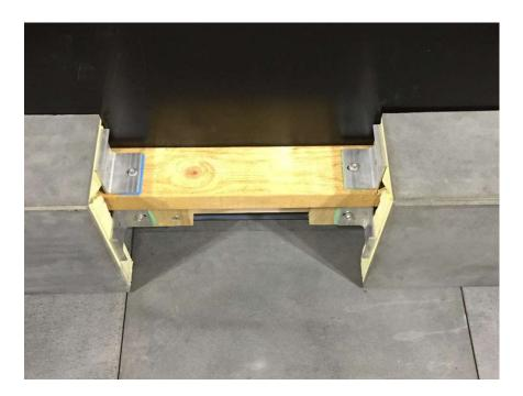
58) The final blocks forming the soffit should be cut exactly to size and preassembled to form the 'quirk mitre' detail, then allowed to cure fully. Once this is done the backing board on the vertical part must be cut to allow the block to be slid into position along the horizontal locating grooves without being fouled by the vertical brackets. Prior to installation sealant should be applied to the areas that will contact the brackets once in place.
