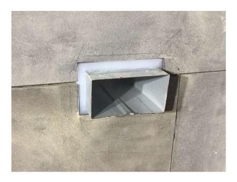
62) Expansion joints and joints between blocks should have a backing rod inserted and be sealed with neutral cure silicone or polyurethane. It is suggested that a complementary colour be selected for all visible joints.
