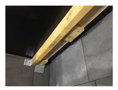
51) Once a block is cut to produce the same 'quirk mitre' detail as described previously along one edge a bracket is pushed into the locating groove prior to installation.
