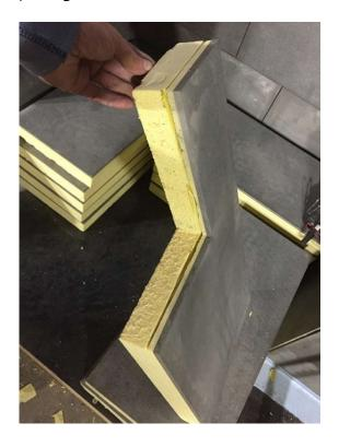
33) Any groove that is cut over size on site should be filled with silicone or polyurethane sealant prior to installation to ensure it fits snugly to the locating flange on brackets and extrusions.
