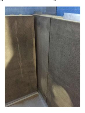
15) Each long run should be started by laying the exterior corners first to set the height. Lines may be run between these corner blocks. It is advised that one or two blocks be laid against the corner blocks before lines are set to help support it and prevent its being moved by the tensioned line.
