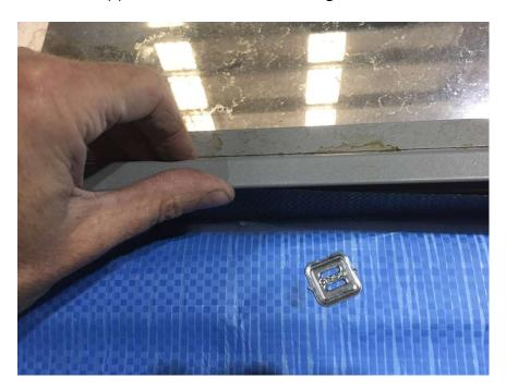
24) The Reveal Rail extrusion may be fixed below a window or door to support a SmartStone Systems sill, and may also be used vertically to close off the cavity beside the window as seen to the right of the window in the picture below.
