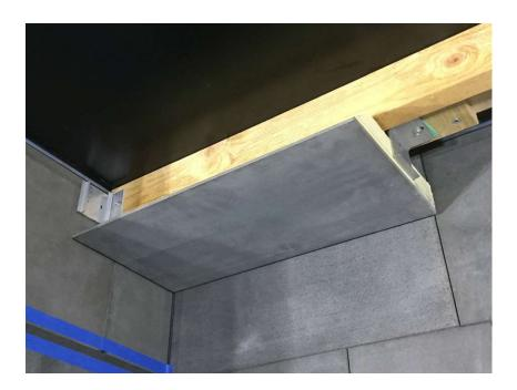
53) It is useful to mark the line of the soffit and vertical elements to help positioning of the brackets.
