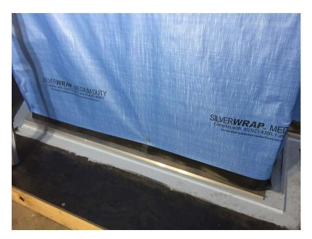
5) All joints in sarking should be lapped a minimum of 50mm and taped.
