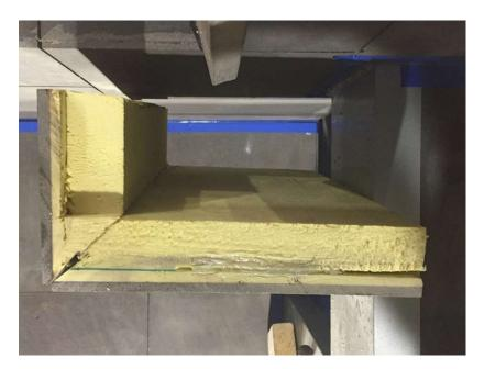
59) An 18mm thick block should be fixed to the frame and adhesive sealant applied to it and the vertical bracket flanges. The block will provide additional support to the vertical block.
