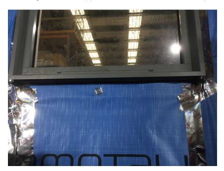
6) The first block is placed on the reveal extrusion so the locating fin sits in the groove in the backing board. PVC or aluminium joiner extrusions are inserted in vertical joints with maximum 10mm spaces between them
