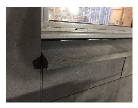
47) Once installed sealant should be inserted between the flashing and the back of the sill to ensure water cannot be blown up and over the back of the sill.
