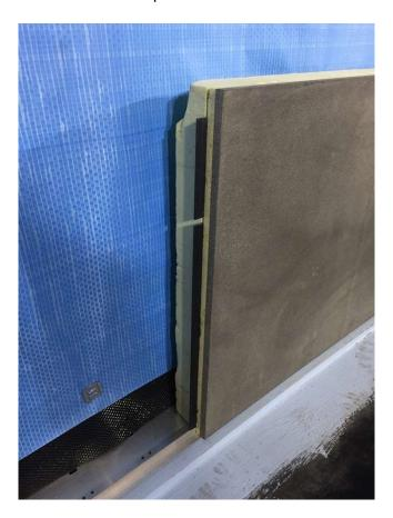
7) Neutral cure silicone or polyurethane sealant is applied between all vertical and horizontal joints before the next block is laid taking care to bridge any gaps between the joiners and clips.
