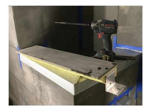
56) The vertical block is then fixed into place and the internal angle may be caulked in a complementary colour to complete the 'quirk mitre' joint.
