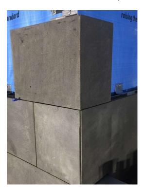
10) To make the quirk mitre detail the end of the block is cut back on a 45 degree angle a set distance from the face. Once one block is laid sealant is applied to the surface adjoining the second block.
