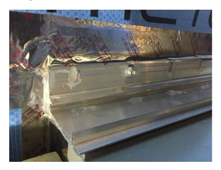
32) Blocks that are to go over the top of windows or doors must have grooves cut into them to accept the locating flanges on the Reveal extrusion both across the top and down the side of opening.
