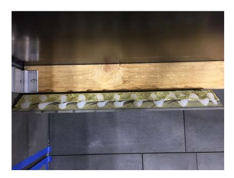
55) Prior to installation of the vertical adjoining piece a bracket is fitted into the locating groove. A tip is to ensure you have your fixing ready to go before you place the block.
