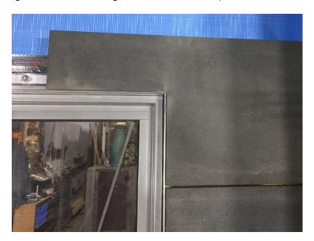
36) Should horizontal expansion joints be required or where blocks must be fitted up to an eave the clips may be used in vertical joints. At the ends short sections of wall up against block work or other adjoining cladding materials the Reveal extrusion may be cut to act as a starting clip as shown on the right in the image below.
