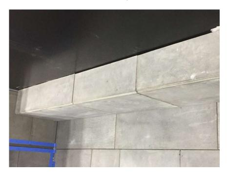
61) Ensure that all penetrations should have had backing rod inserted and are sealed.
