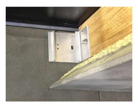
54) Once the horizontal elements are installed silicone or polyurethane sealant is applied to the surface of the backing board that will meet the adjoining vertical block.
