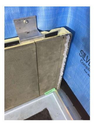
14) Where expansion joints are specified for structural purposes a 10mm gap is left that must have backing rod inserted before being filled with flexible sealant.
