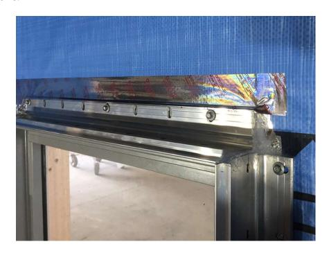
31) All screw holes, fixings and all weep holes on the Reveal extrusion used as a lintel over an opening must be filled with silicone to ensure water tightness. Note that above meter boxes and other penetrations that do not have self-draining design features a 5-10mm gap should be left between blocks and extrusions that must then be filled with backing rod and sealant.
