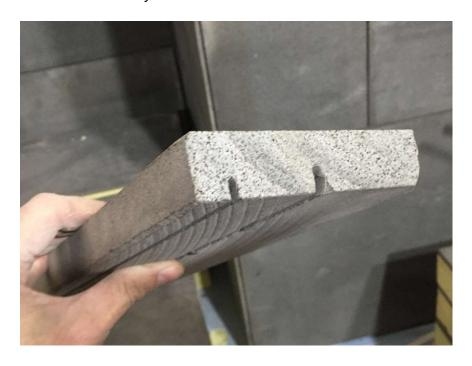
45) Before placing the sill in position, a bead of silicone or polyurethane sealant should be applied along the locating groove, and a few spots on the support ledge at the back of the Reveal extrusion. The support ledge the sill is set at an angle of 10 degrees.
