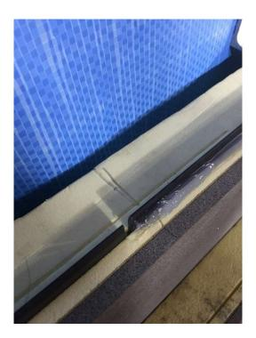
17) Sarking should wrap parapet walls completely into box gutters, lap onto penetrations such as windows and meter boxes, and tape used to seal joints in sarking and to all penetrations.
