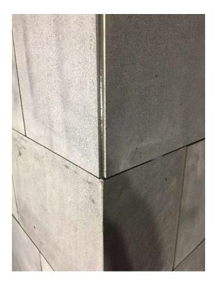
13) Internal corners should have the blocks overlapped and sealant applied in vertical joints.
