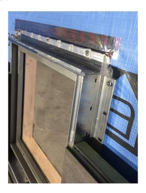
35) Once installed should any sealant squeeze out of joints as the block is installed it is best left to go hard before being cut back with a sharp knife.
