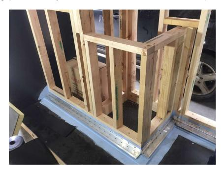
3) Once the Reveal Rail extrusion has been fitted dampcourse is fixed to the frame ensuring that the bottom edge extends below the level of the fixing screws.
