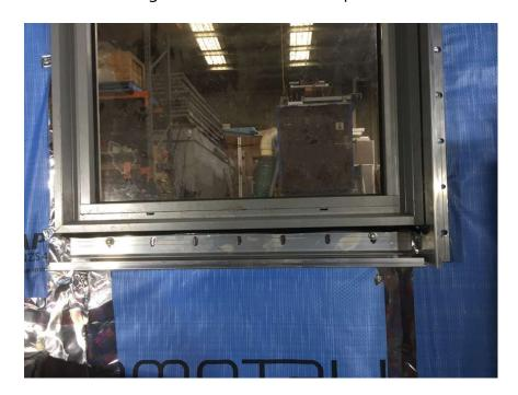
25) The same extrusion may be used as a lintel above the window. The junction between the vertical and horizontal extrusions should be closely fitted with the horizontal lintel above the vertical reveal as seen below.
