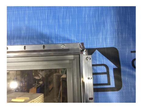
26) There a block runs below a window is should be cut to fit underneath the Reveal extrusion that will support the sill. A groove must be cut into the vertical part of the cut to accept the locating flange on the Reveal extrusion that runs up the side of the window.
