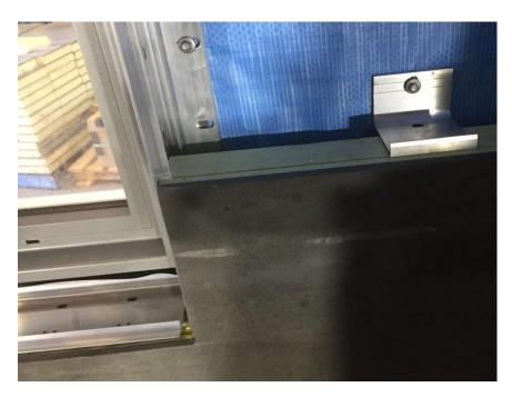
30) Tape should be applied to the top edge of the Reveal extrusion that forms the lintel, and the junction between the vertical and horizontal Reveal extrusions sealed with silicone.
