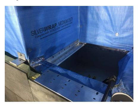
20) Flashings over parapet walls are required to ensure water tightness of the wall.
