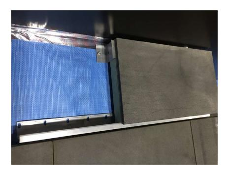
42) Joiner extrusions and silicone or polyurethane sealant is to be applied to fill the vertical joint.
